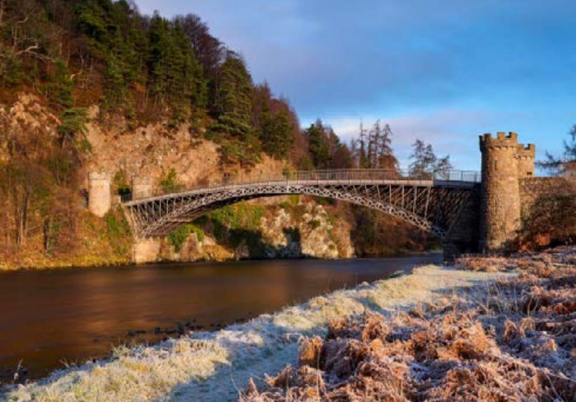
Thomas Telford's latticed cast iron Craigellachie Bridge, spanning the Spey, with two sets of mock-medieval crenelated towers standing 15ft (4.5m) high on each side of the river.
